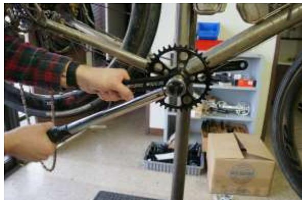
Fig.8 Torque to 50 Nm.
