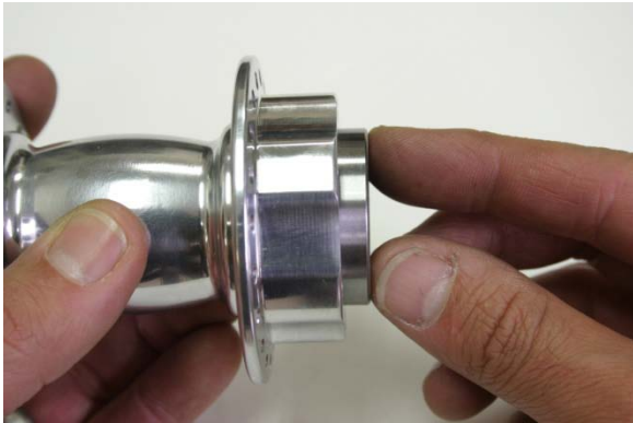
Fig.8 Make sure bearing goes straight into bore.
